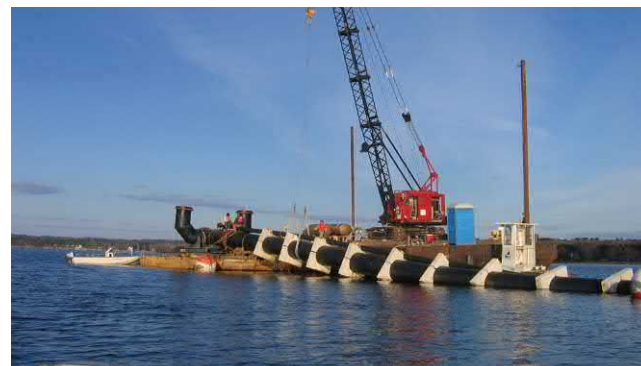
Raw Water Intake Pipeline – South Burlington, VT
