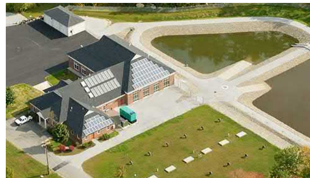
Microfiltration Membrane Facility – Rockport, ME
