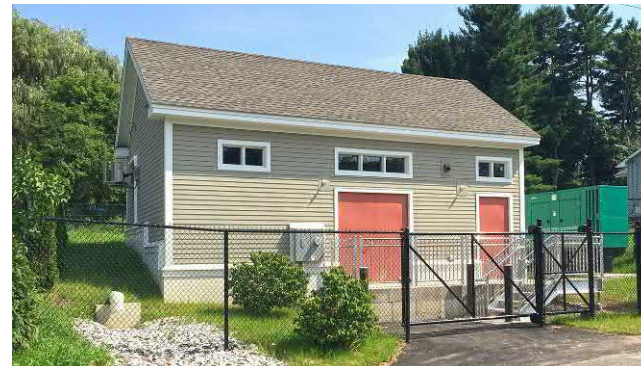
Booster Pump Station – Bethel, CT
