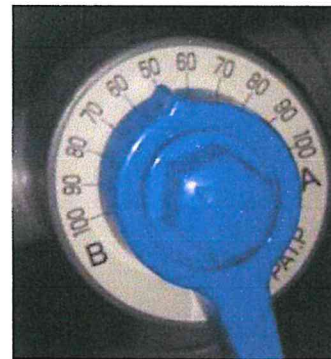
At start-up, and for standard operation, the Aeration Balance Control Valve (blue) should be set to 50%.
