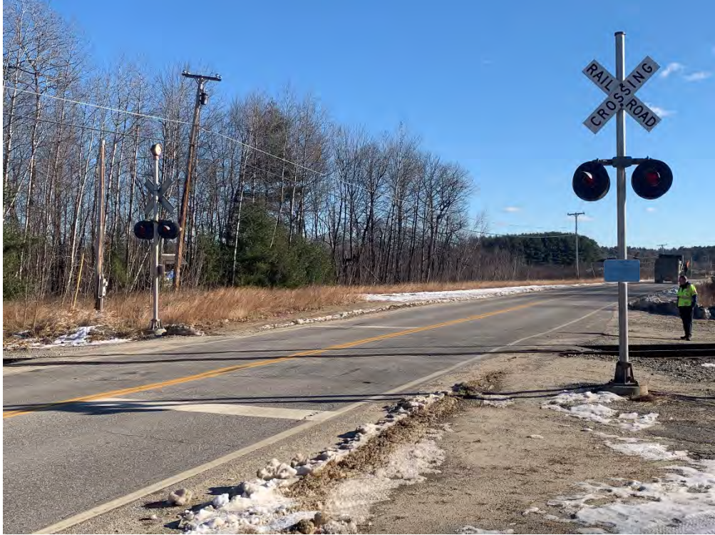
MP 172.10 – New Gloucester Rd Crossing
