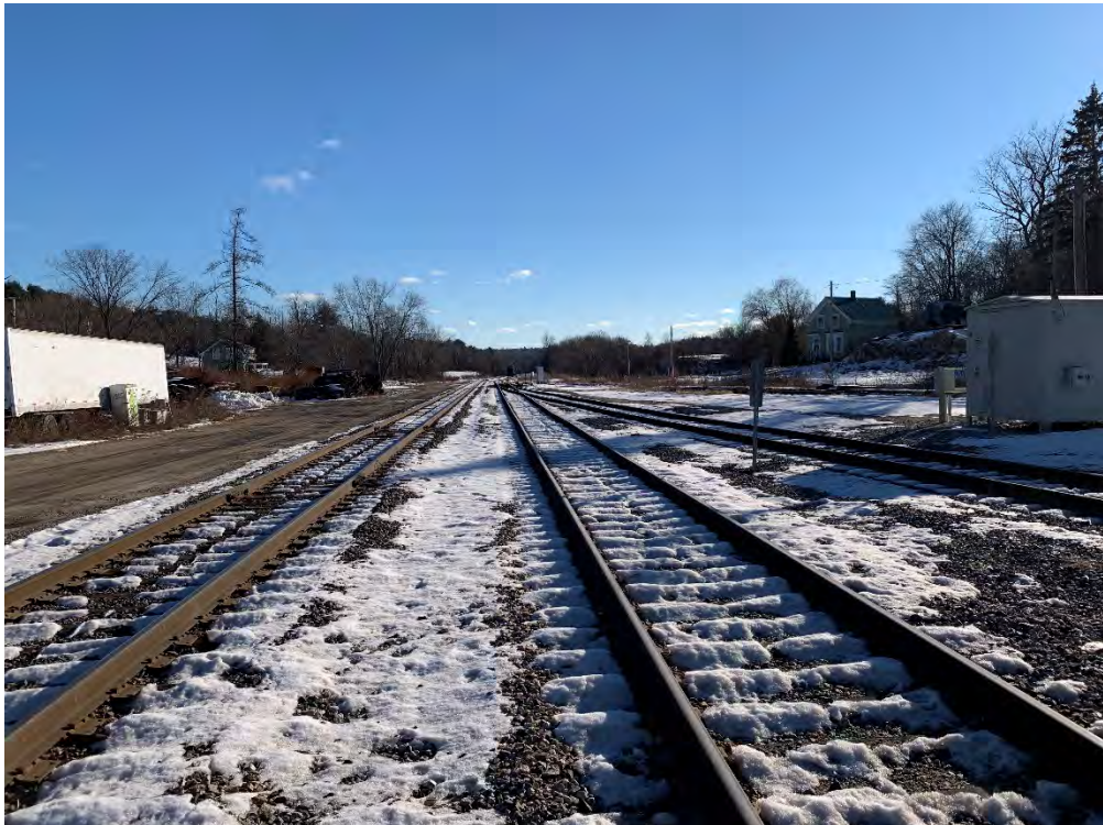
MP 167.60 – Danville Junction Yard East End
