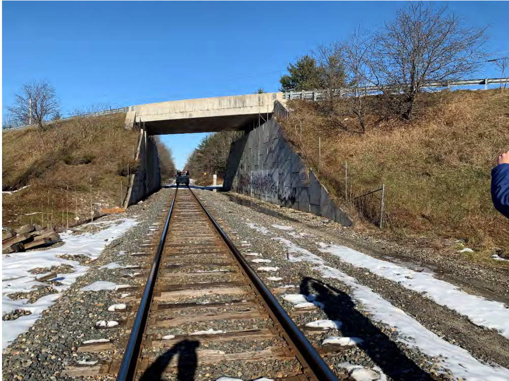
MP 182.08 – Sligo Rd Bridge
