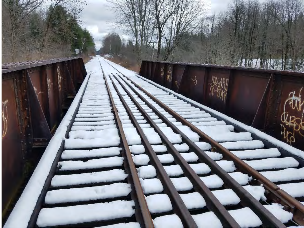
MP 24.90 – Royal River 2 nd Bridge
