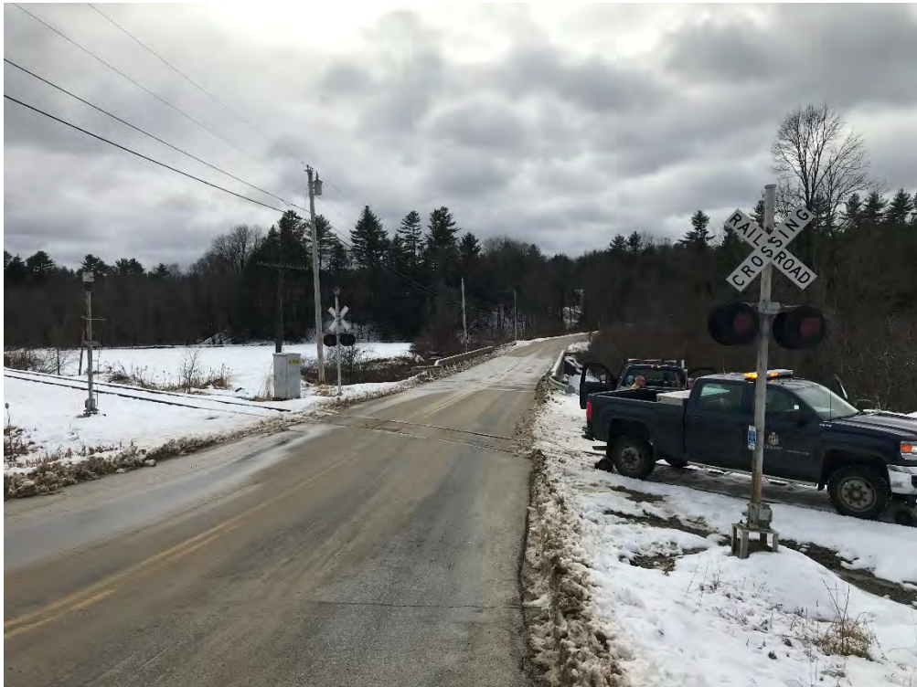
MP 24.55 – Cobbs Bridge Rd Crossing
