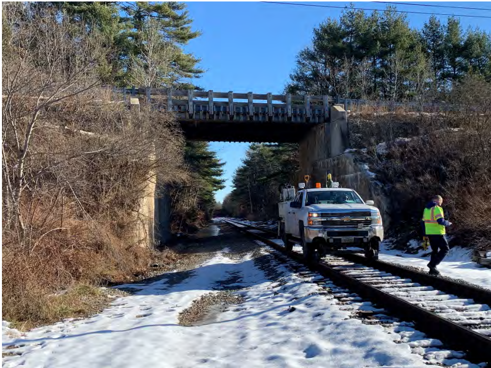
MP 180.01 – New Gloucester Rd Bridge
