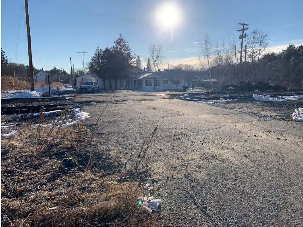
MP 160.05 – Libbys Ave Industrial Crossing
