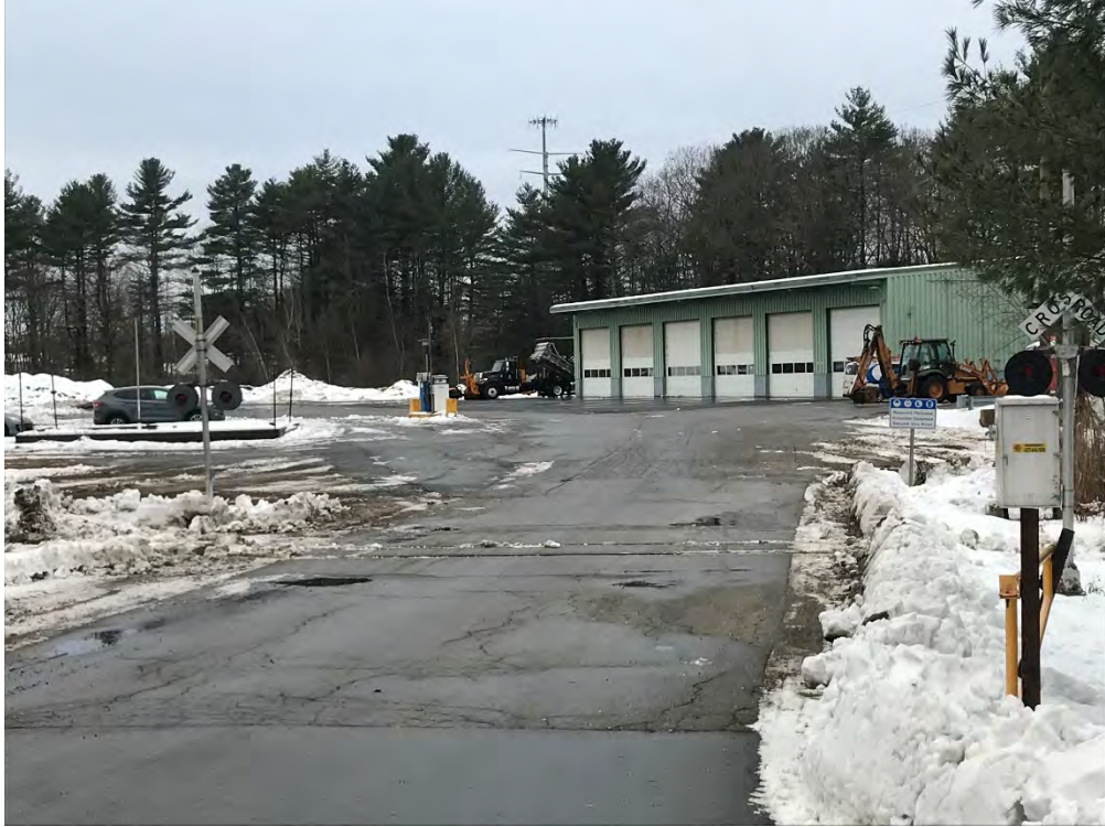
MP 10.14 – State Garage Crossing
