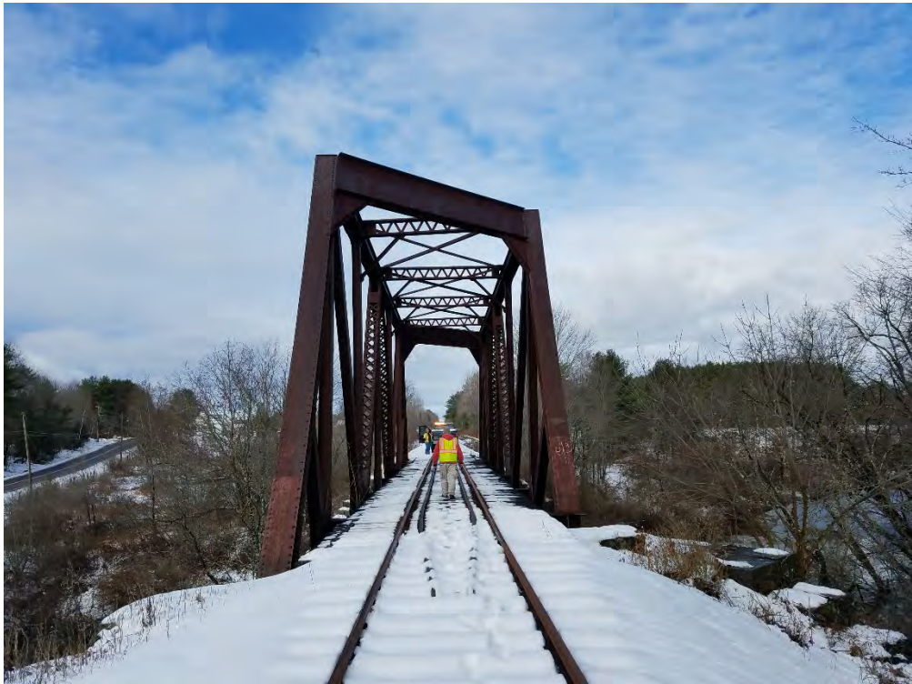
MP 15.70 – Royal River 5 th Bridge
