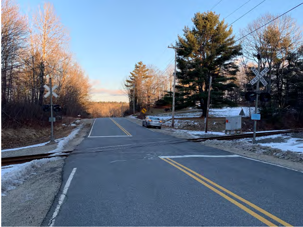
MP 178.80 – Mill Rd Crossing
