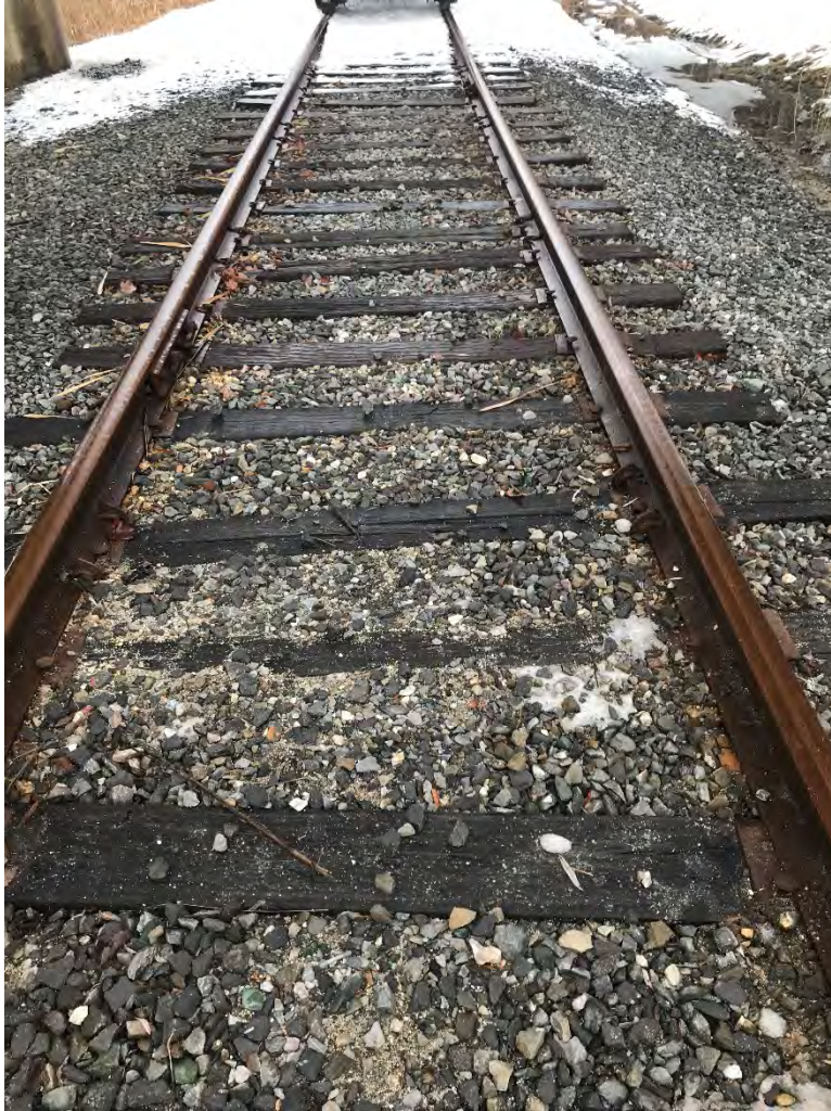
MP 8.99 – Tuttle Road Bridge
