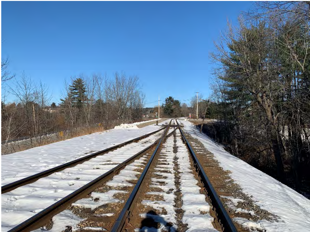
MP 166.95 – Danville East Switch
