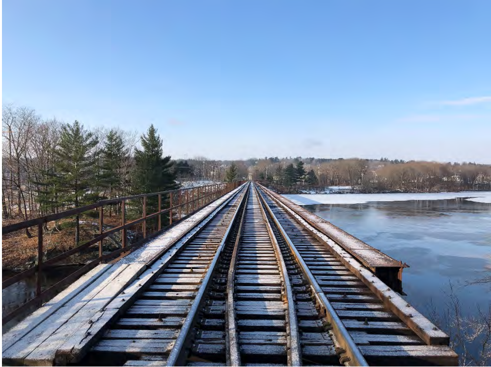
MP 161.22 – Androscoggin River Bridge
