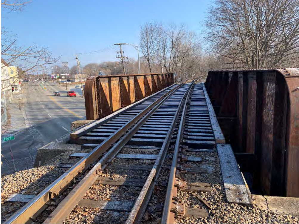
MP 161.43 – Turner St Bridge
