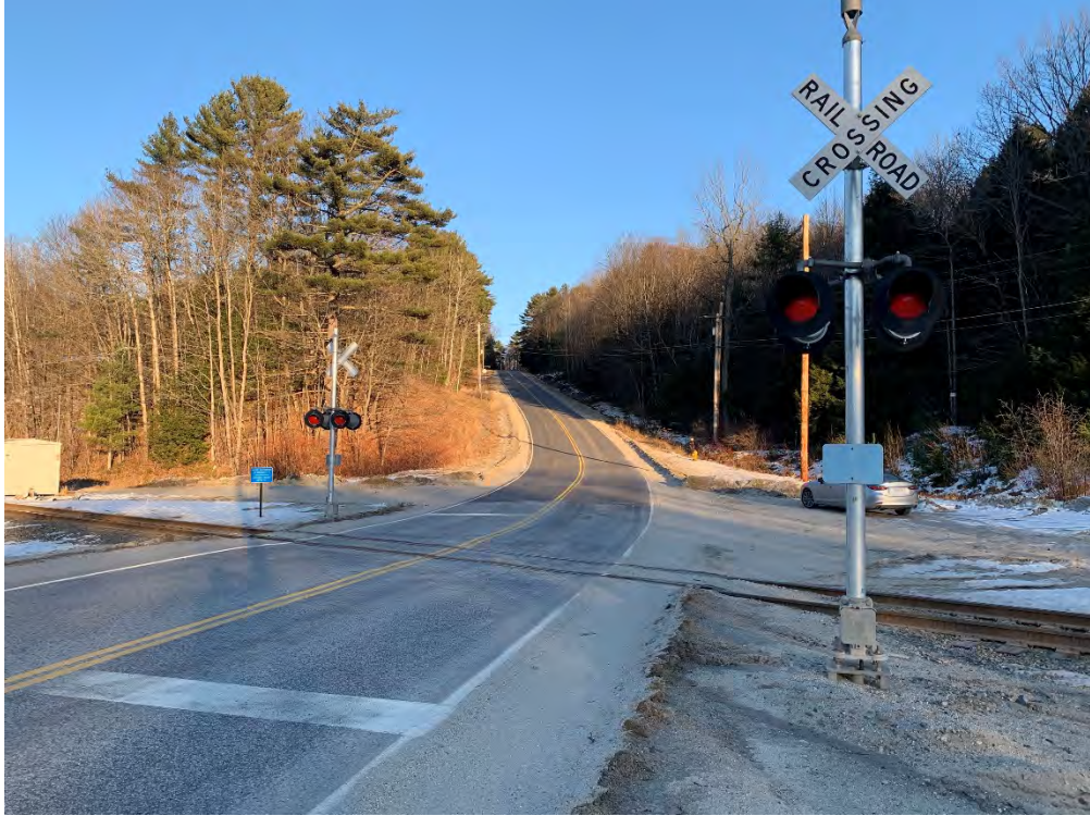
MP 176.73 – Depot Rd Crossing
