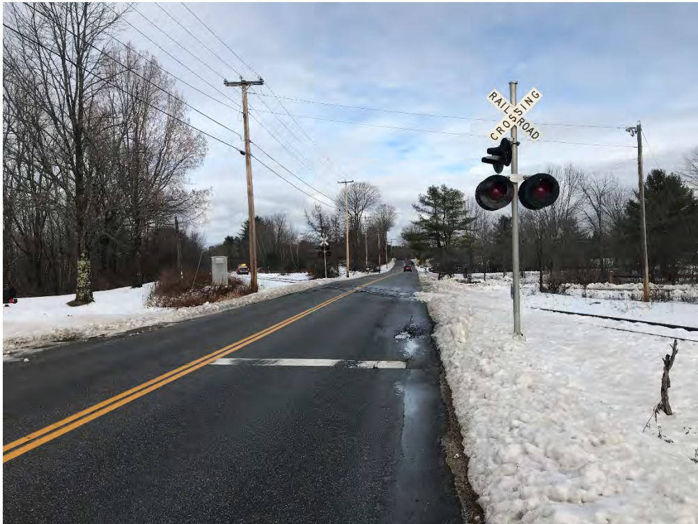
MP 14.89 – Sawyers North Rd Crossing
