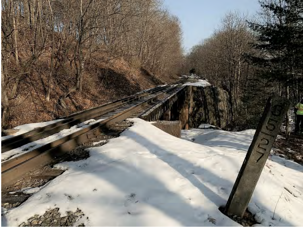
MP 162.73 – Grand Trunk Railway Bridge
