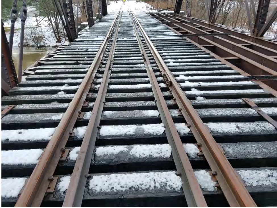
MP 11.66 – Royal River 6 th Bridge
