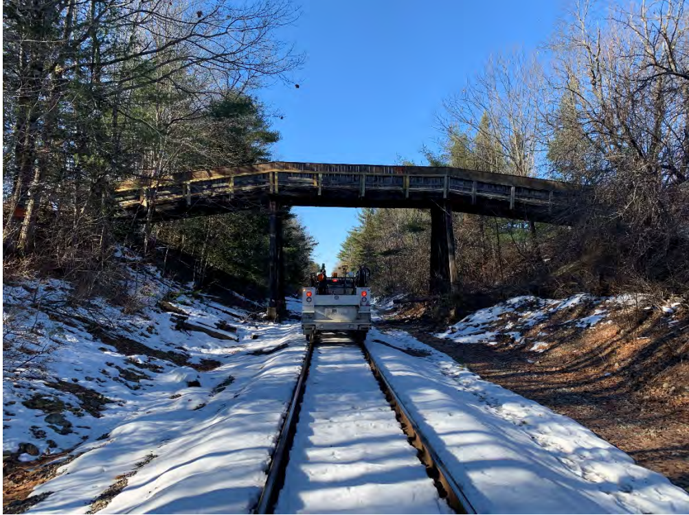
MP 180.37 – Hayes Farm Rd Bridge
