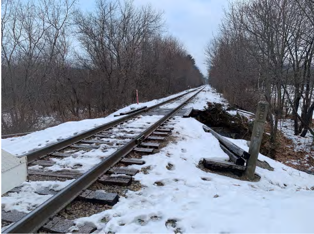
MP 158.92 – Barkers Bridge
