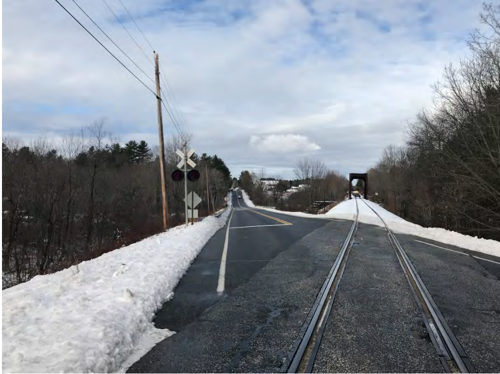
MP 15.60 – Atkinson Bridge North Rd Crossing
