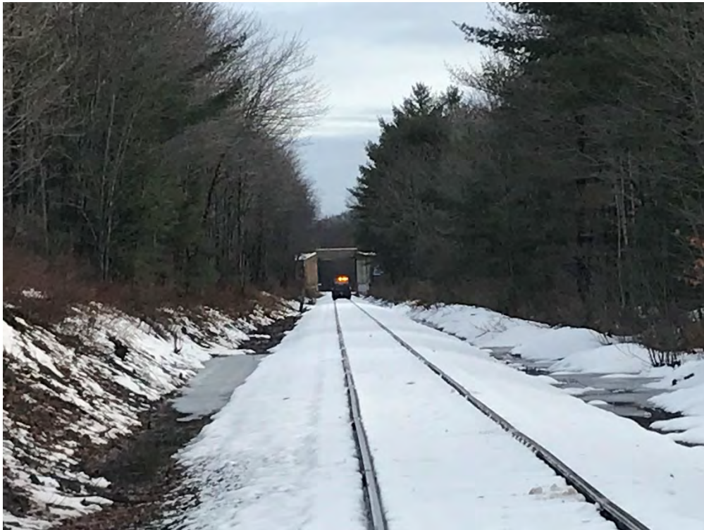
MP 5.95 – I95 Bridge
