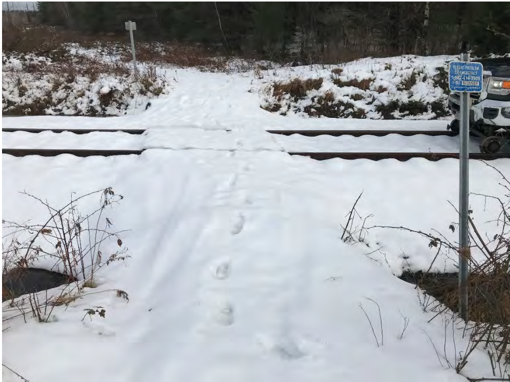
MP 18.01 – Farm Utility Crossing
