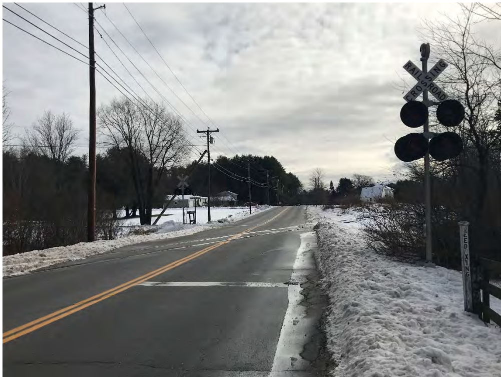
MP 14.17 – Skillings North Rd Crossing
