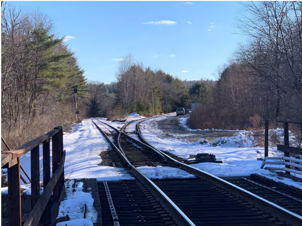
MP 168.05 – Royal River Bridge Junction
