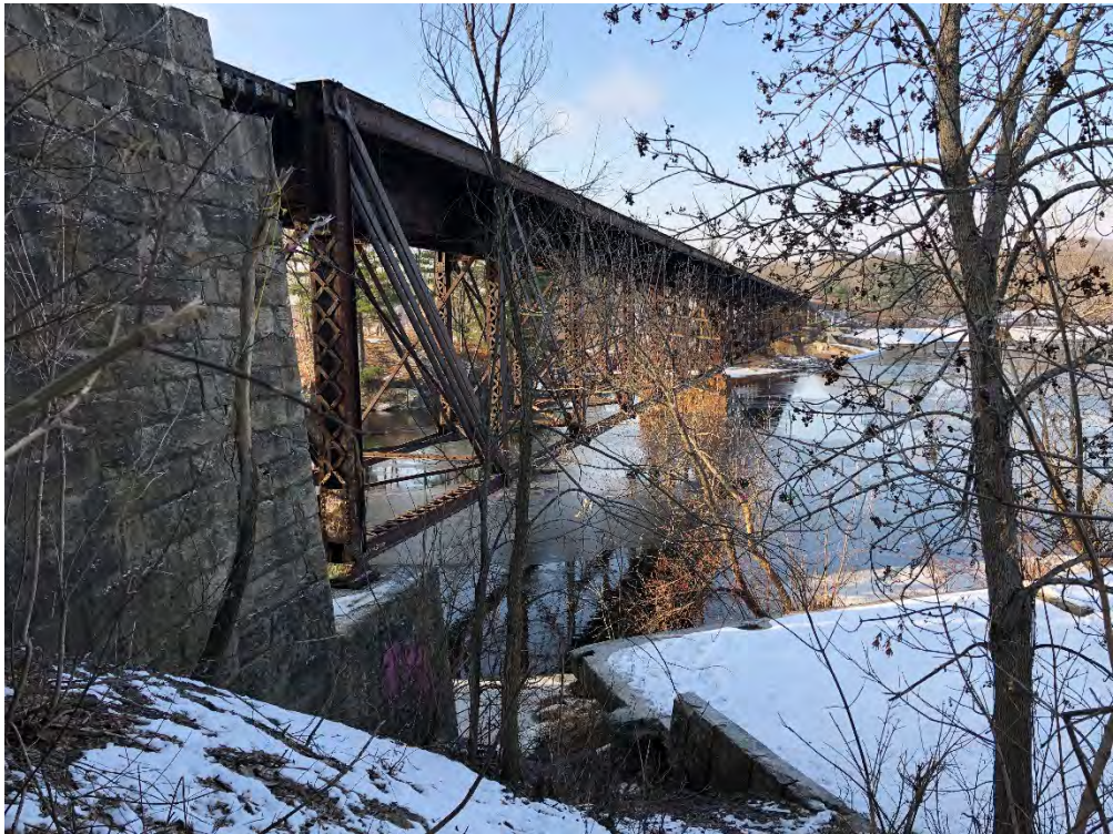
MP 161.22 – Androscoggin River Bridge
