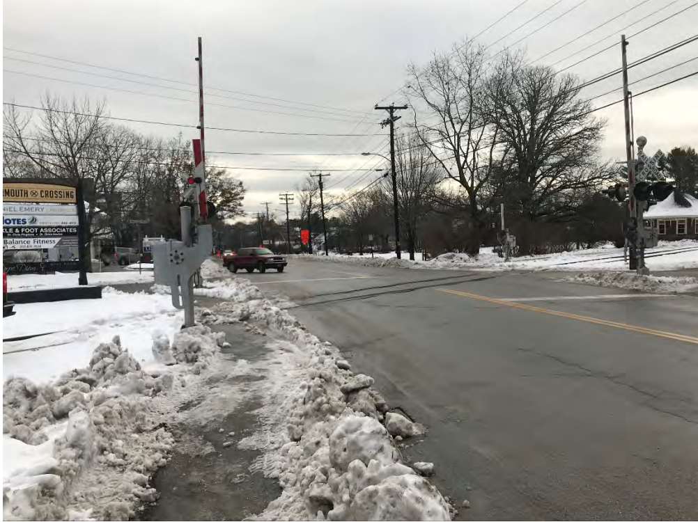
MP 11.34 – Main St Crossing
