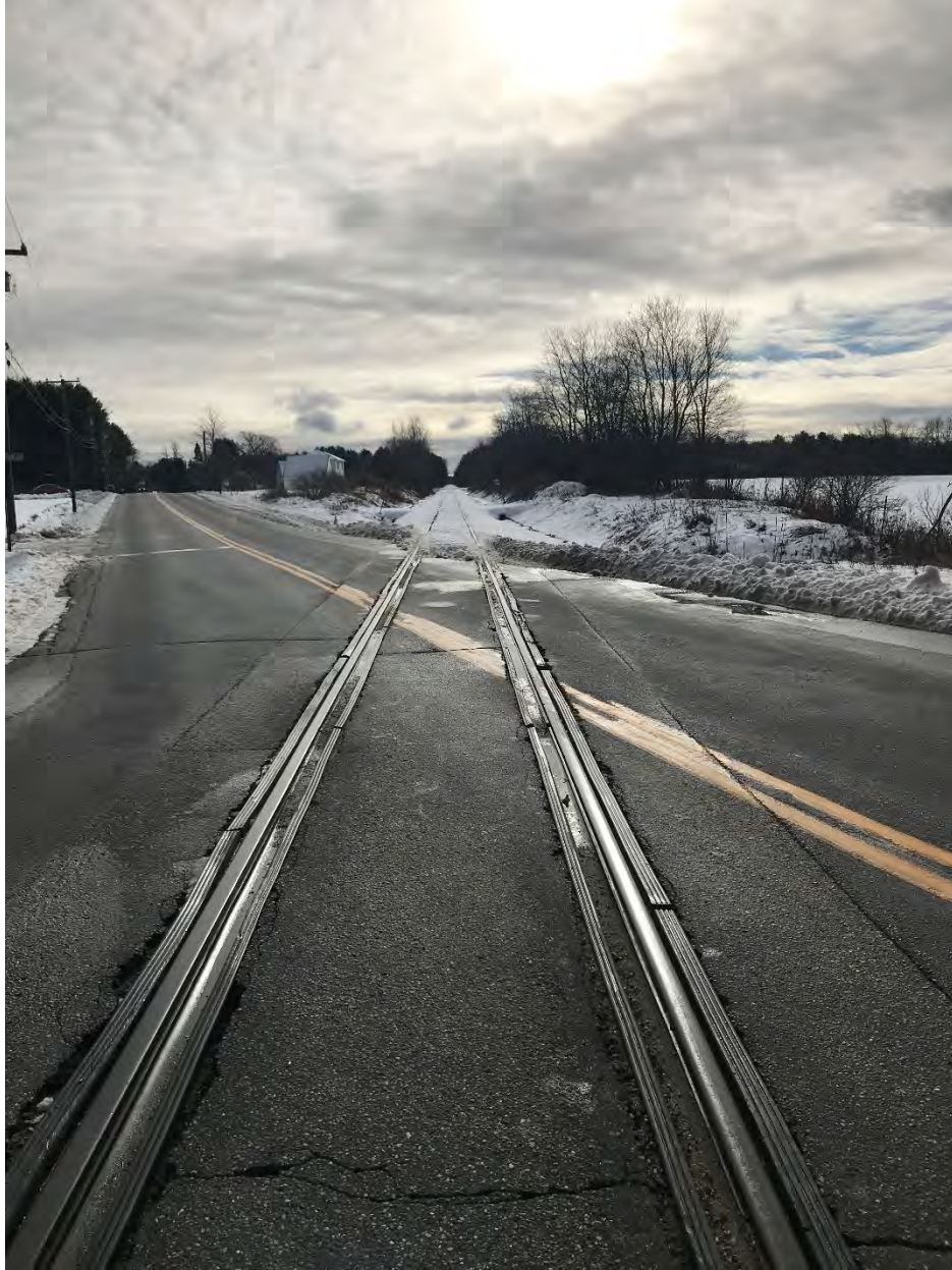
MP 14.17 – Skillings North Rd Crossing
