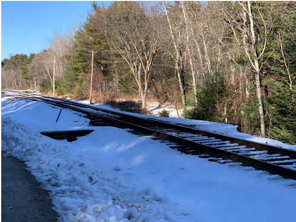
MP 168.20 – 168 West Switch
