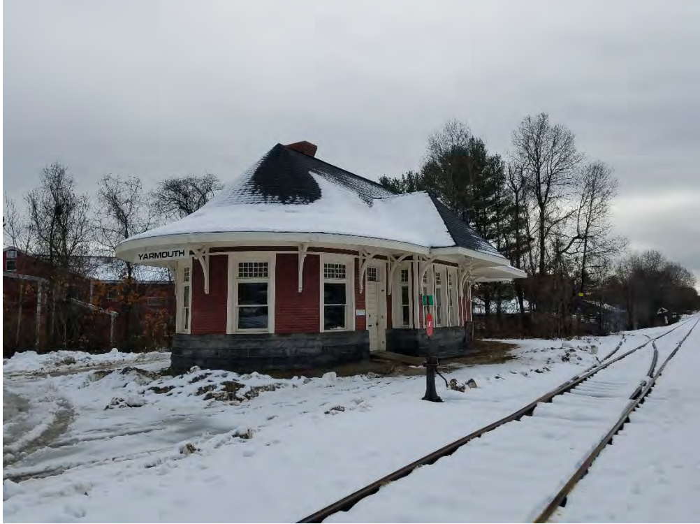
MP 11.2 – Former Yarmouth Station
