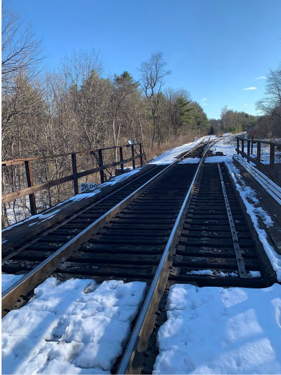
MP 168.05 – Royal River Bridge
