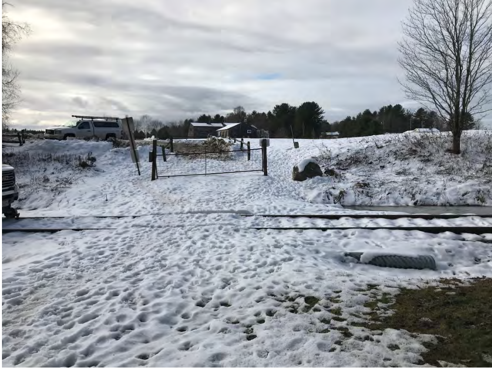
MP 16.06 – Recreation Trail Crossing
