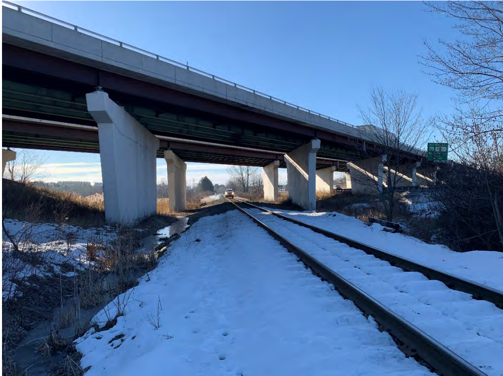
MP 166.09 – I-95 Bridge
