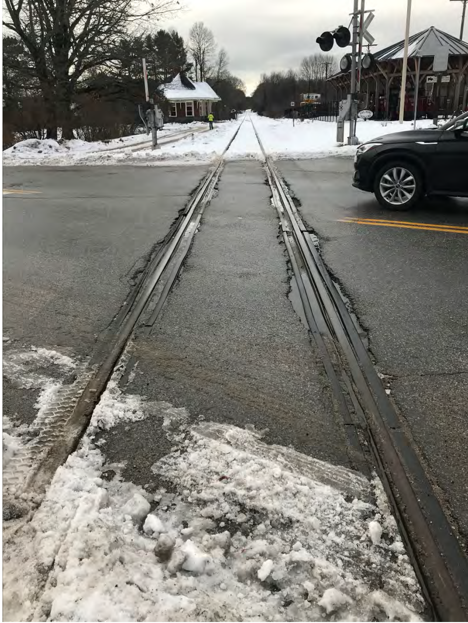
MP 11.34 – Main St Crossing
