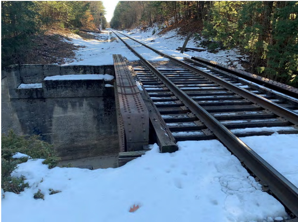
MP 170.54 – Cobbs Rd Bridge
