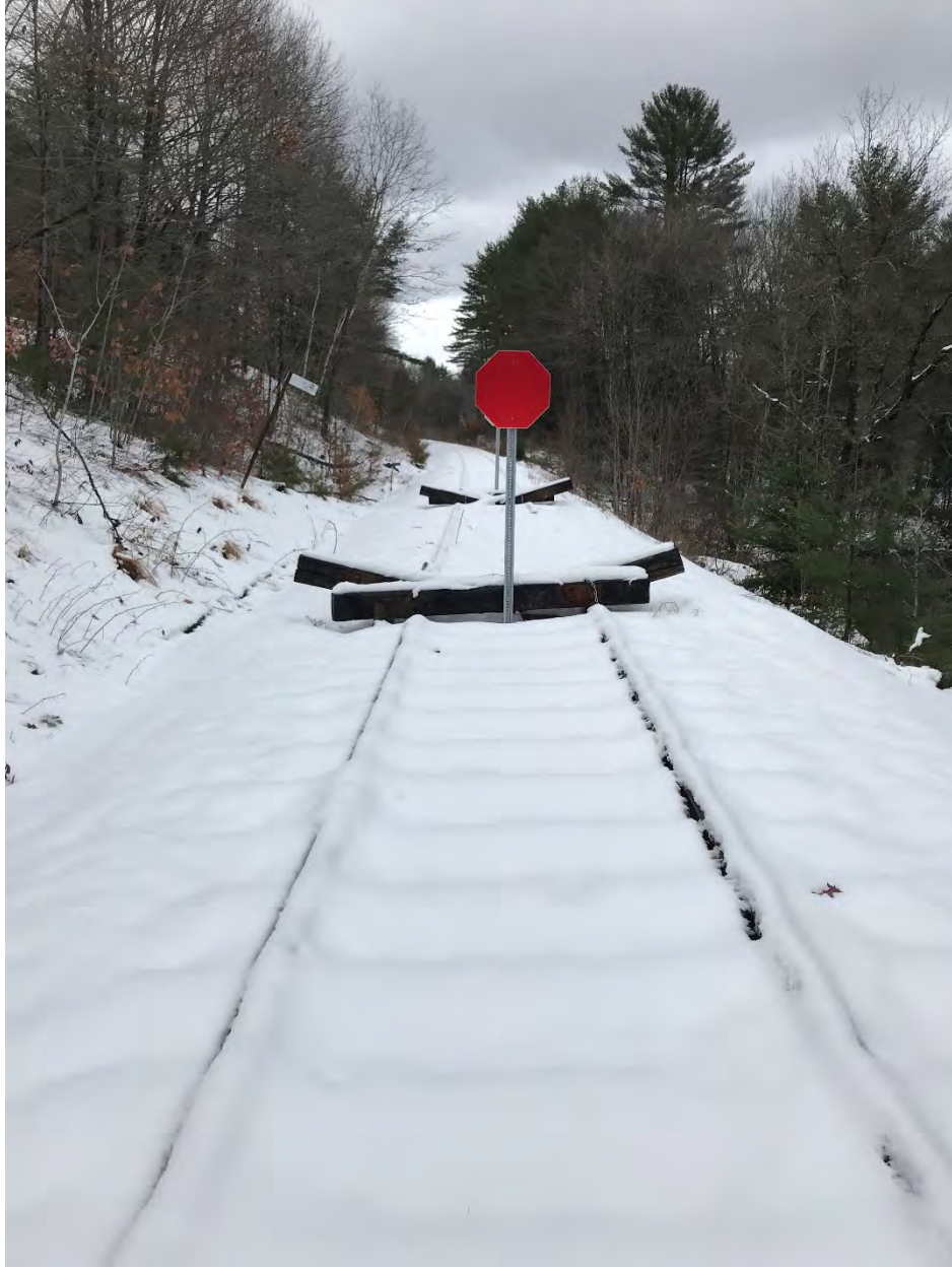
MP 26.0 – MaineDOT Barricade
