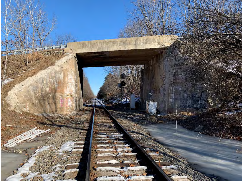
MP 165.88 – Rounds Crossing Bridge
