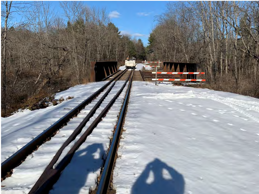
MP 177.16 – Royal River Bridge
