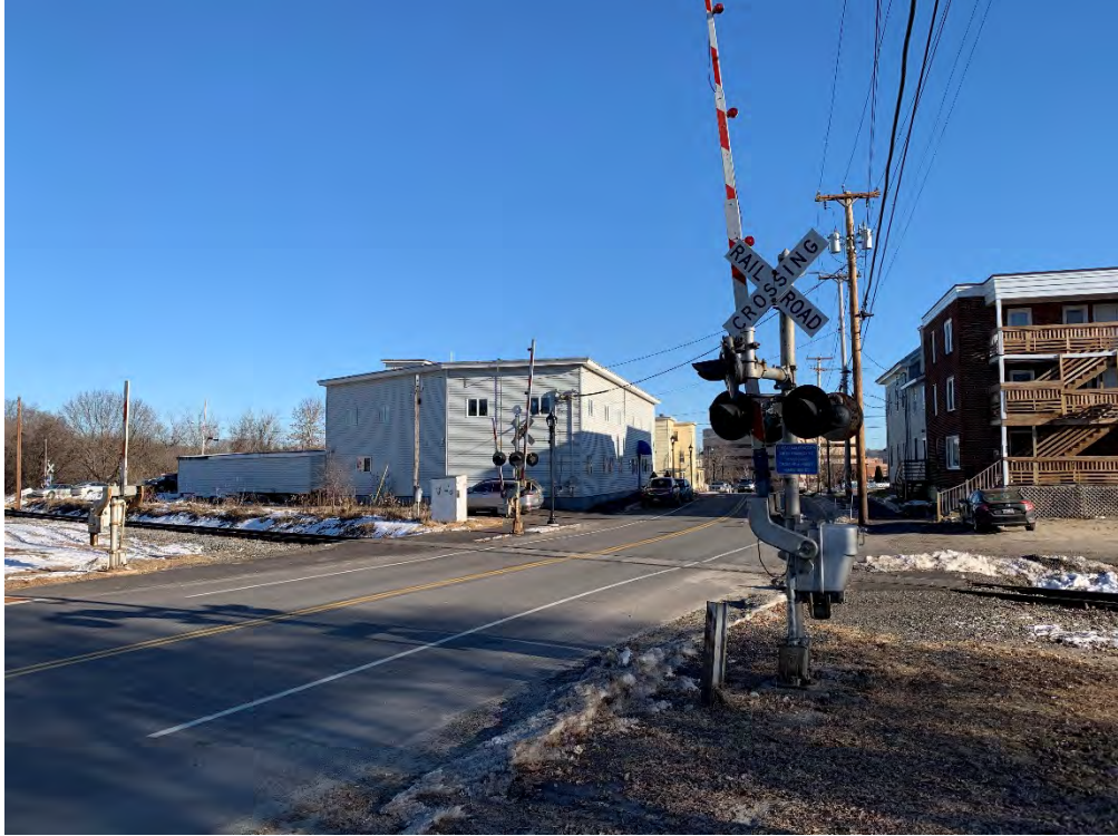
MP 161.55 – Hampshire St Crossing
