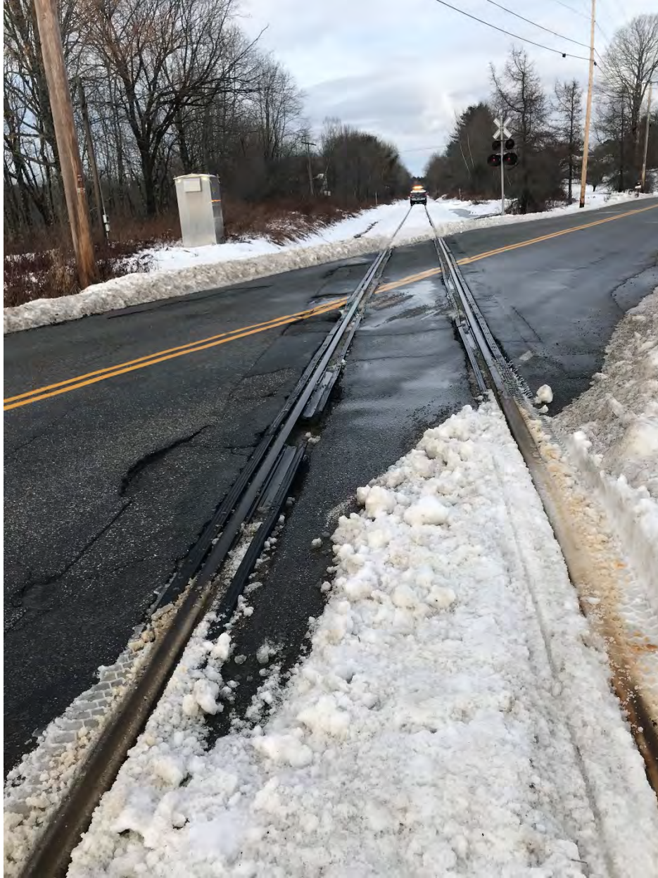
MP 14.89 – Sawyers North Rd Crossing
