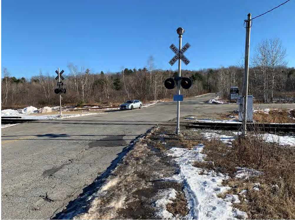
MP 166.19 – Sampsons Crossing
