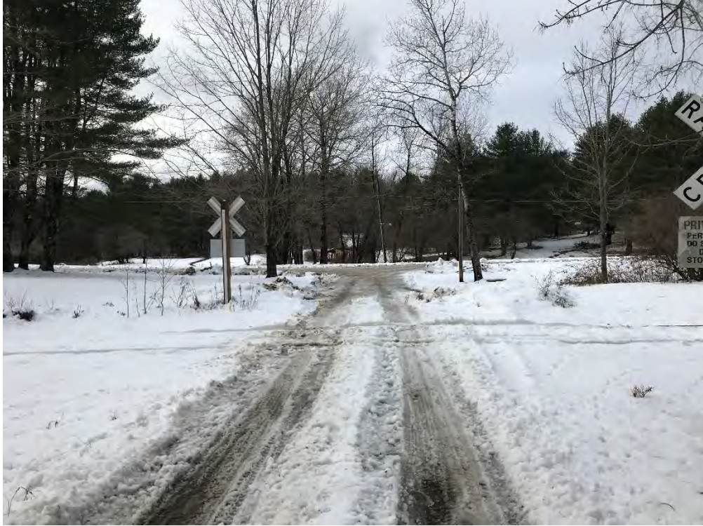
MP 18.54 – Depot Rd Private Crossing
