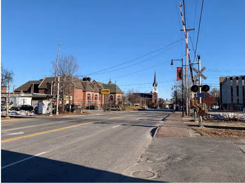
MP 161.67 – Court St Crossing
