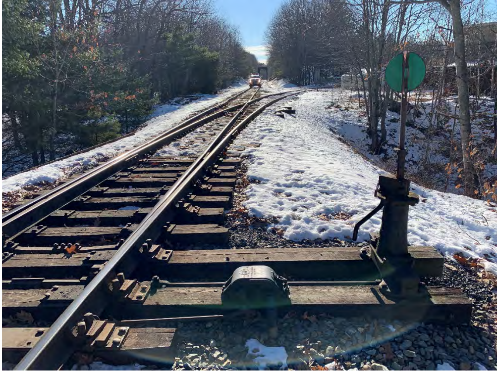
MP 163.60 – Maine Metal Siding
