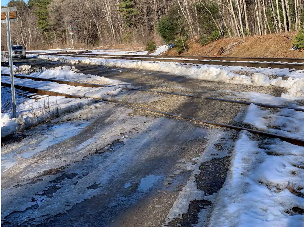
MP 168.15 – Private Maintenance of Way Crossing
