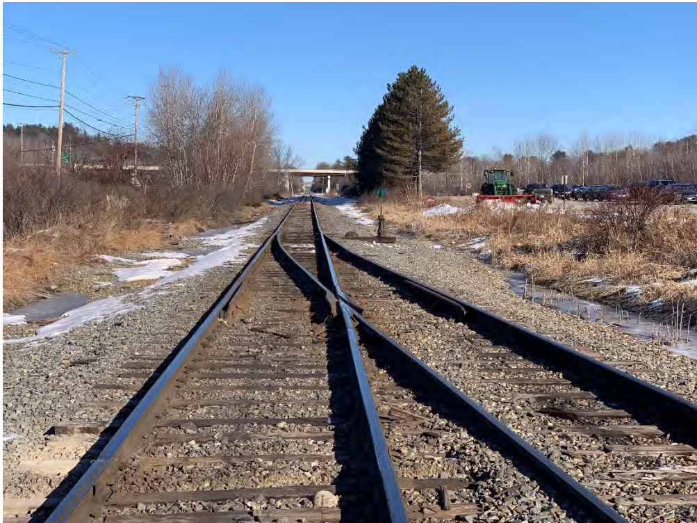
MP 166.50 – International Paper Siding
