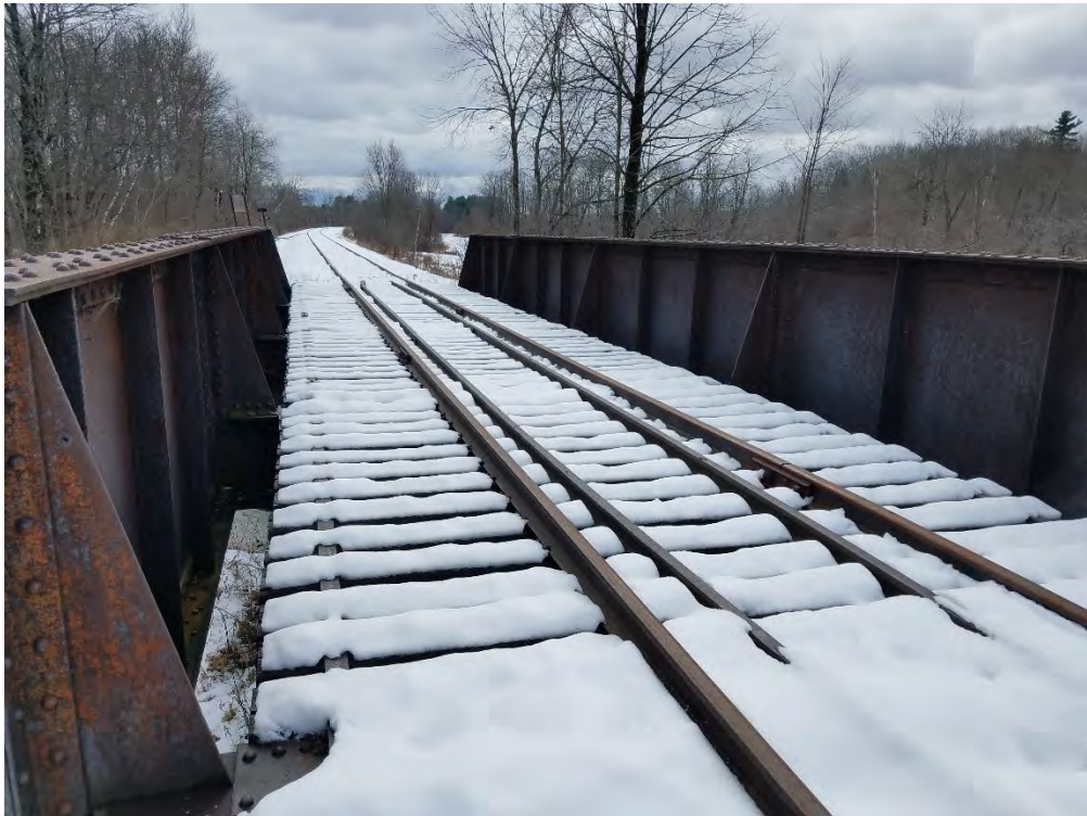
MP 23.90 – Royal River 4 th Bridge
