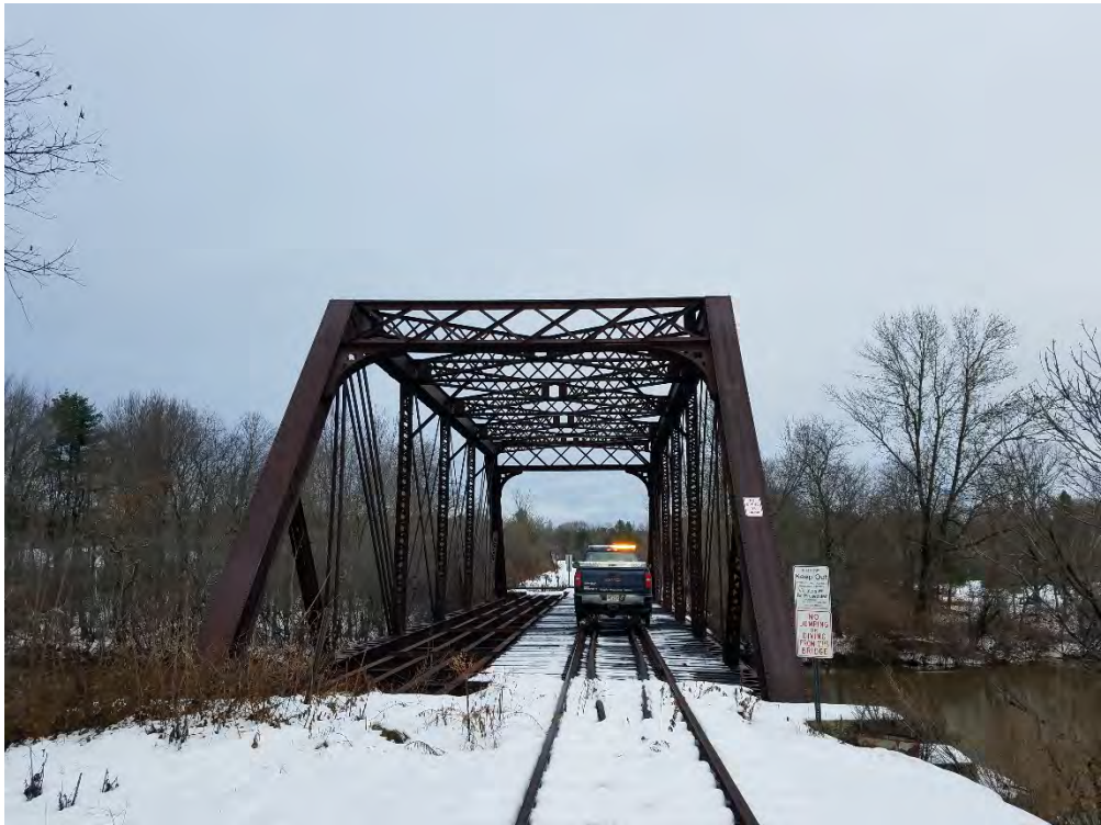
MP 11.66 Royal River 6 th Bridge
