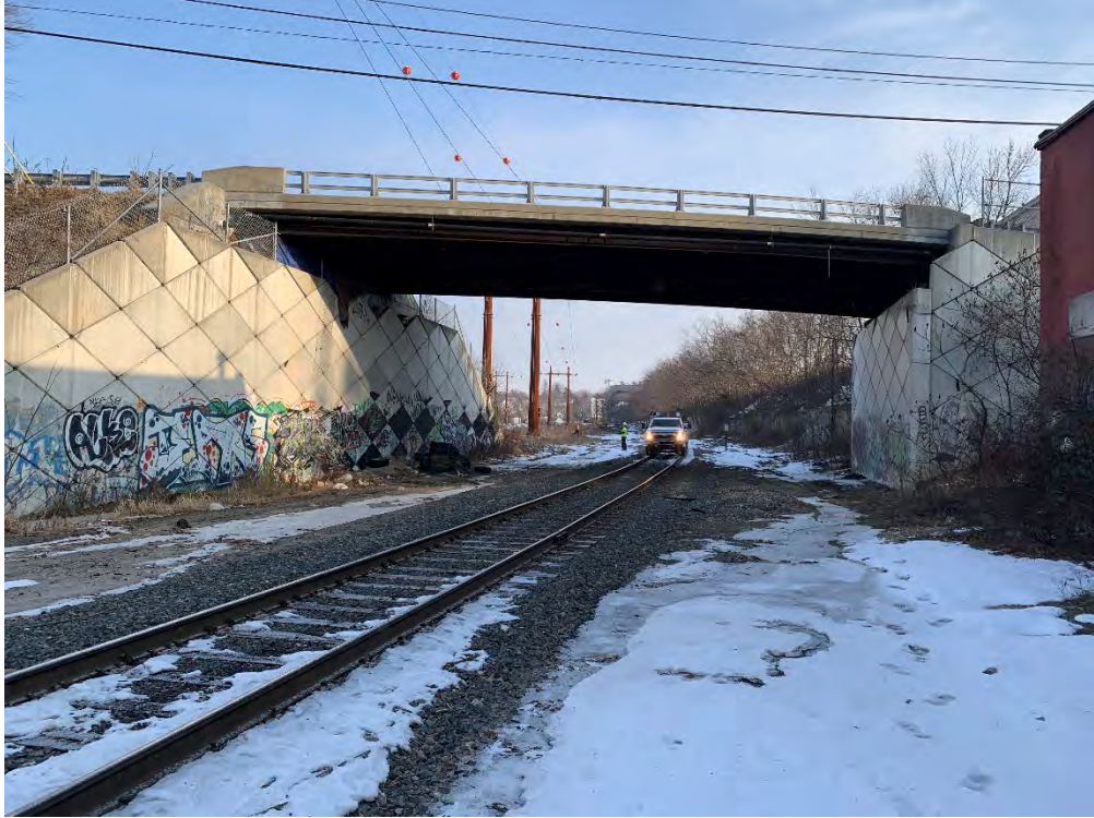
MP 160.88 – Bridge St Bridge
