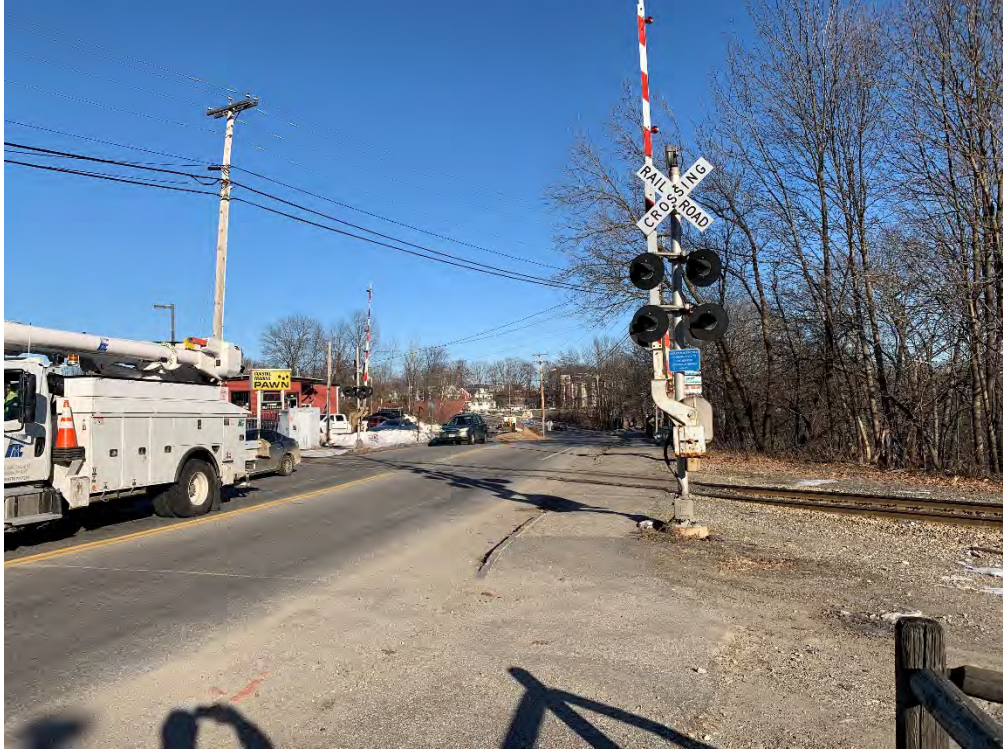
MP 162.15 – High St Crossing
