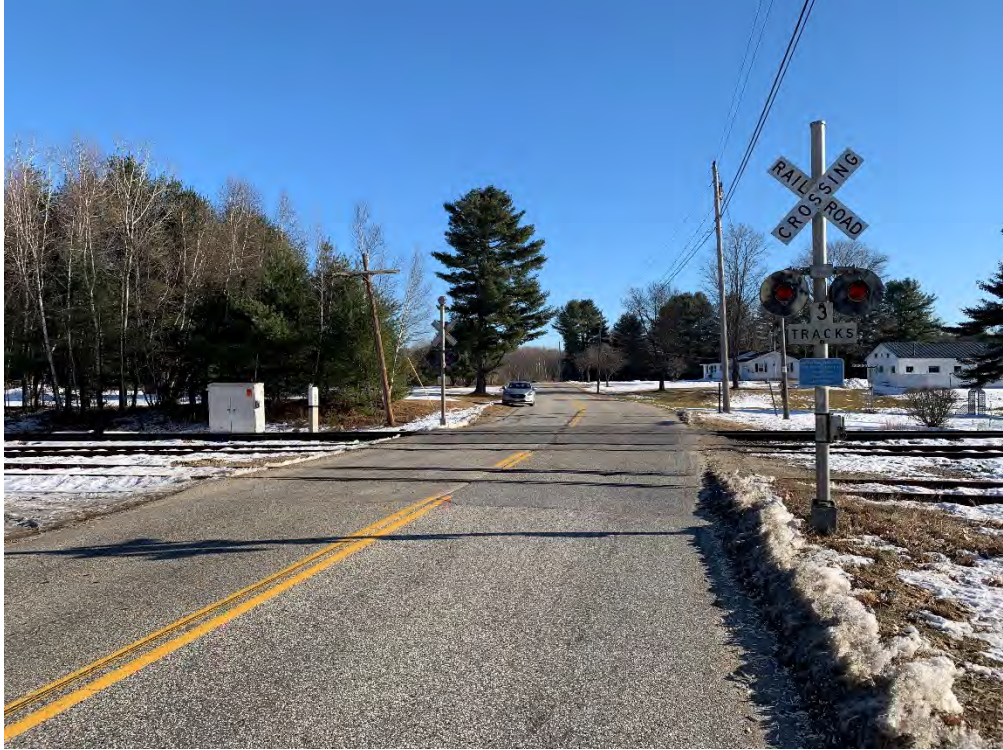
MP 165.00 – Hackett Rd Crossing
