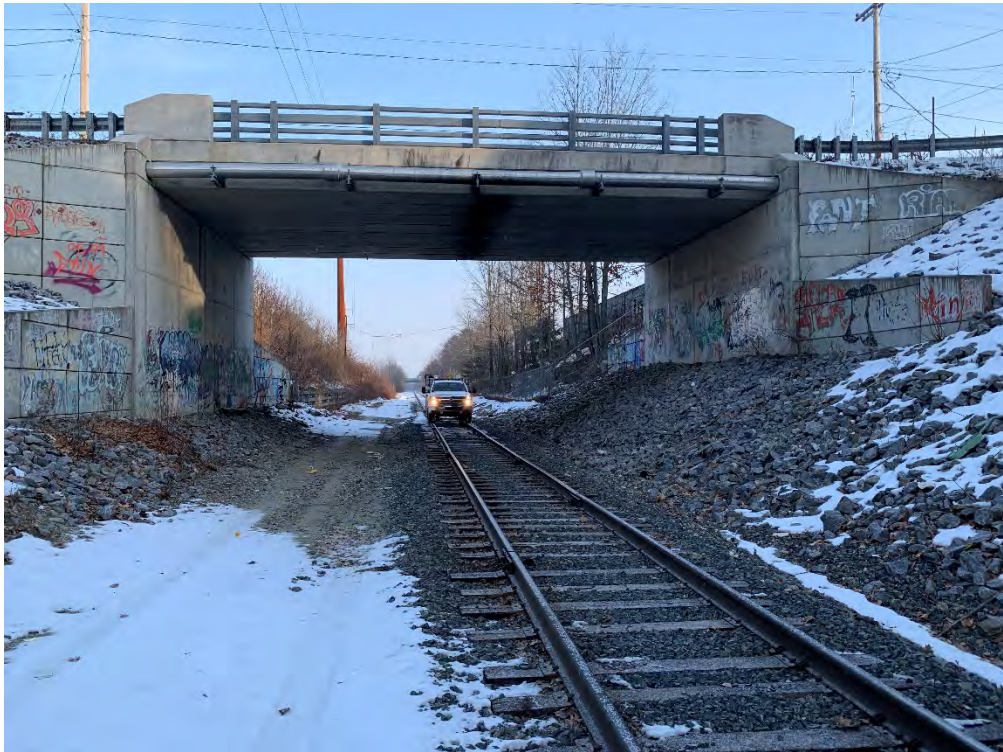
MP 160.44 – Riverside St Bridge
