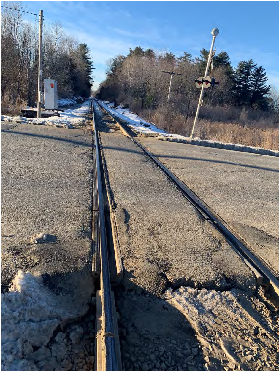
MP 158.42 – Stetson Rd Crossing
