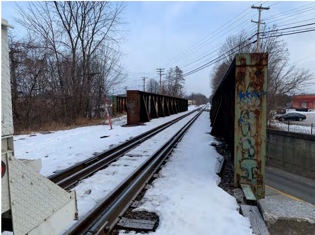
MP 159.18 – Main St Bridge
