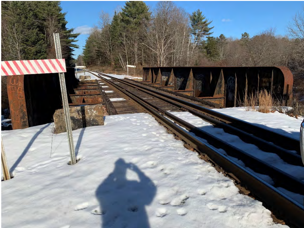
MP 176.14 – Royal River Bridge
