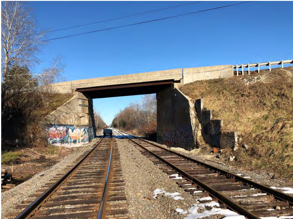
MP 184 – W Main St Bridge
