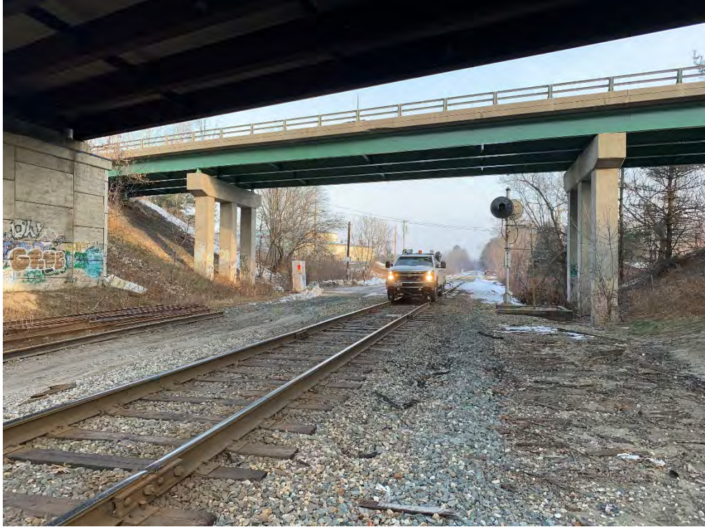
MP 160.08 – Russel St Bridge
