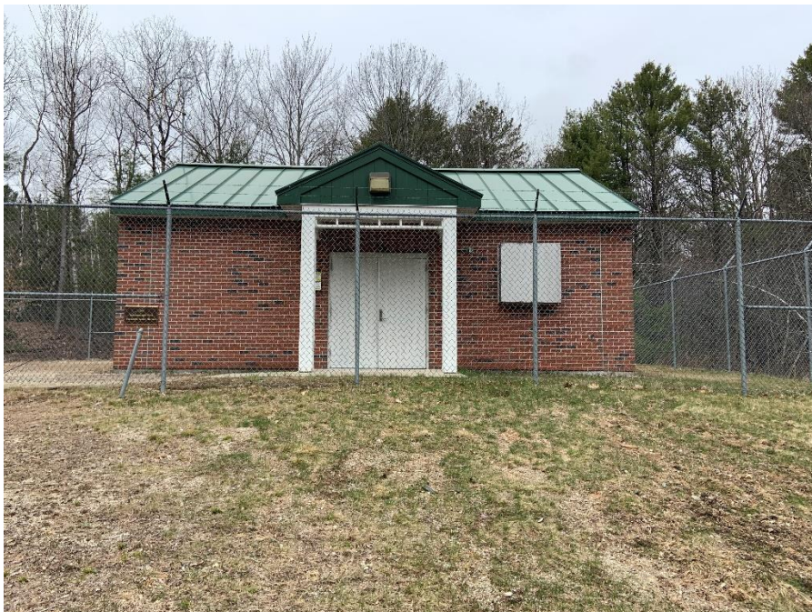
Existing Reinsborough Well building
