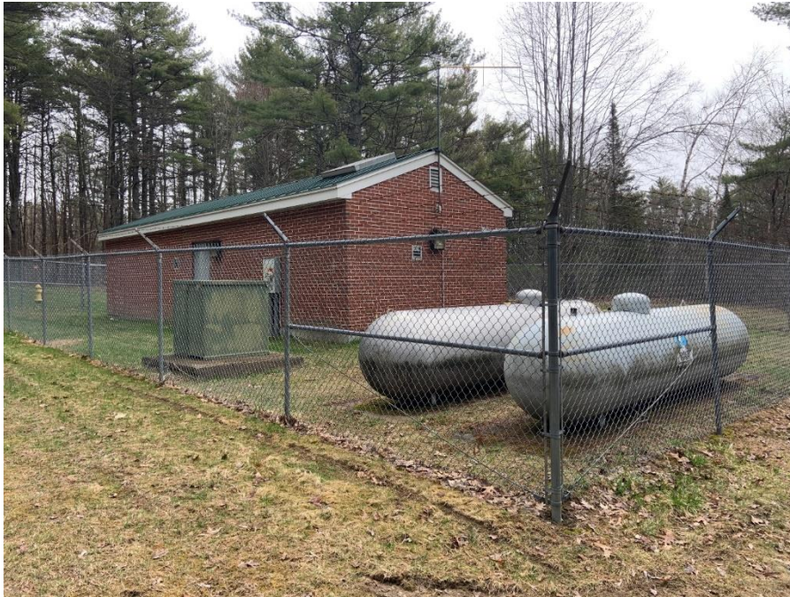
Existing Hayes Well site
