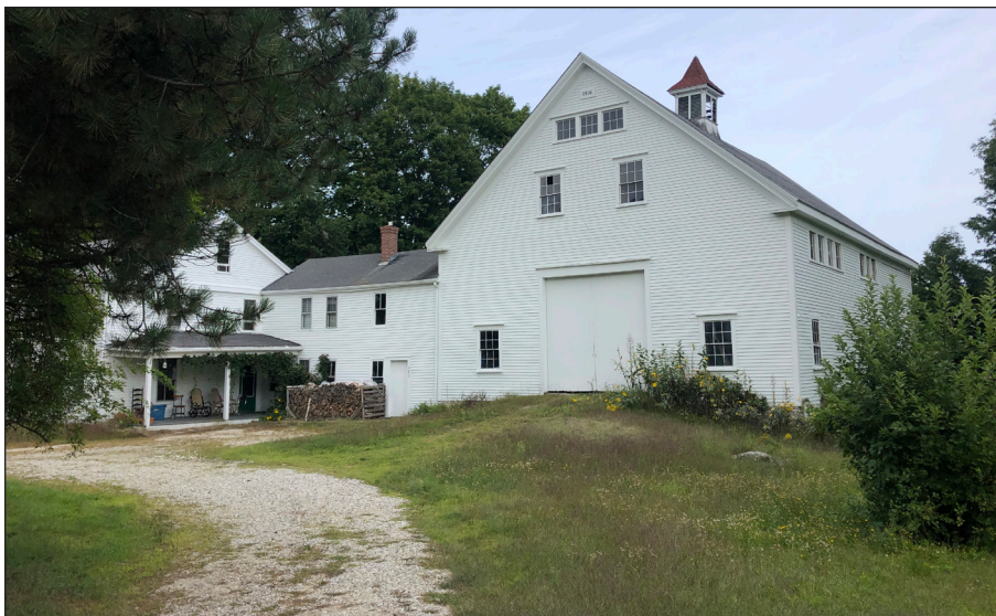
Large historic house and connected barn on Rt 115 near The Lane.
