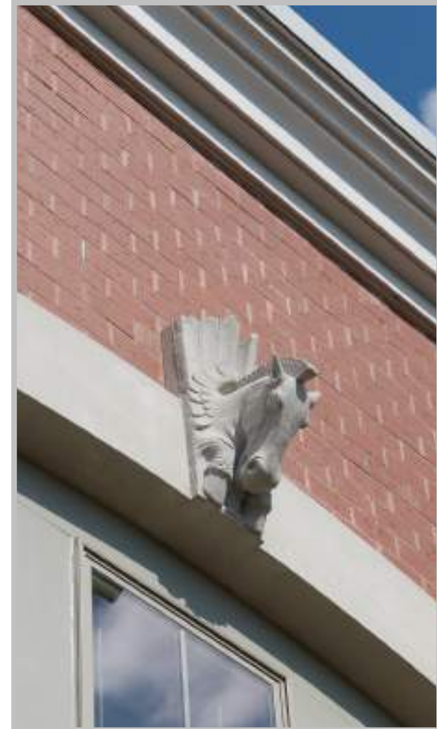
Saco Central Fire Station: The beloved details of horses from the historic Fire Station were incorporated in the new facilities design .
