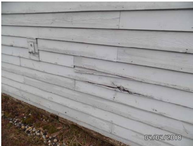
Damaged siding materials were observed in multiple locations on building exterior.
