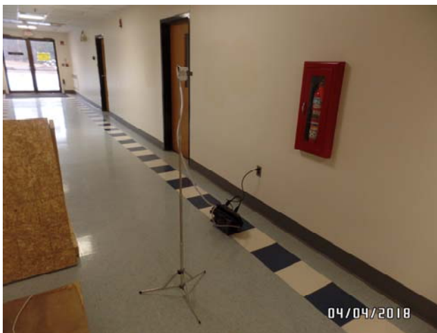
Mold Air Sample (A-3) in corridor near Room #11
