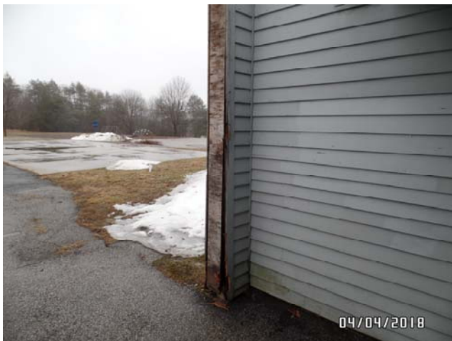
Damaged siding materials were observed in multiple locations on building exterior.
