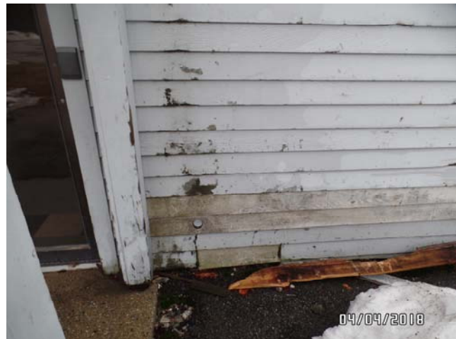
Damaged siding materials were observed in multiple locations on building exterior.
