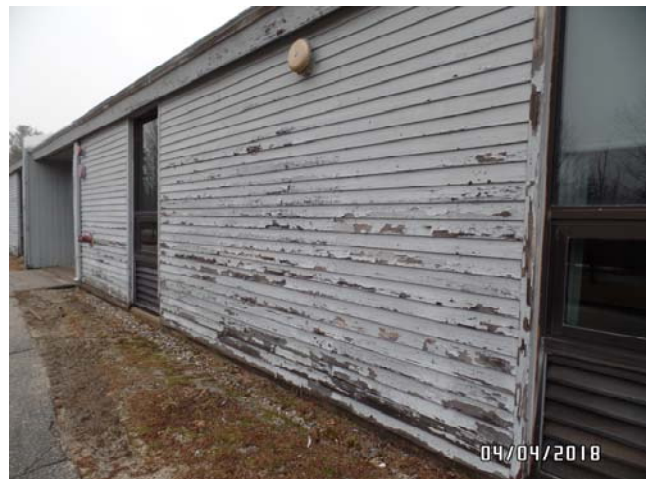
Damaged siding materials were observed in multiple locations on building exterior.
