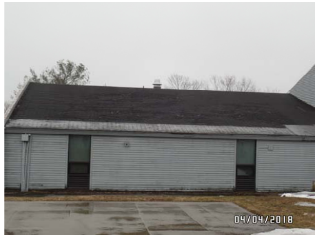
Shingled roofing areas are in need of replacement.
