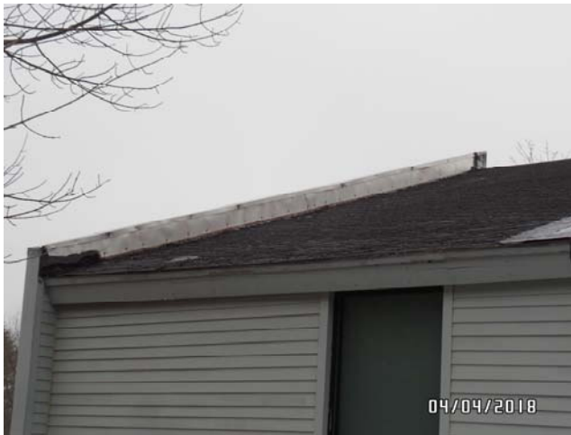
Shingled roofing areas are in need of replacement.
