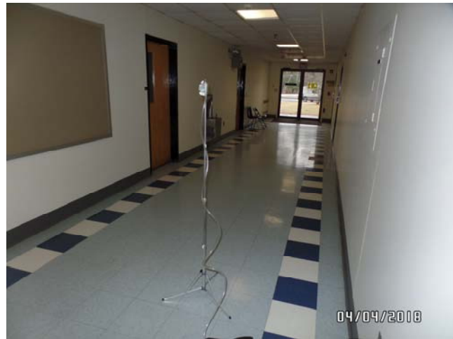
Mold Air Sample (A-2) in corridor near Room #3.
