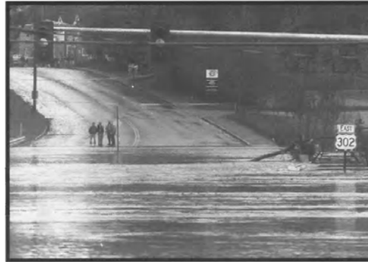
Figure 5. Presumpscot River at Route 302 in Westbrook, Maine (site 11) on October 22, 1996. Note the high-water mark on Route 302 and the debris or the upstream guardrail of the bridge (Photograph by David A. Rodgers, The Portland Newspapers).
