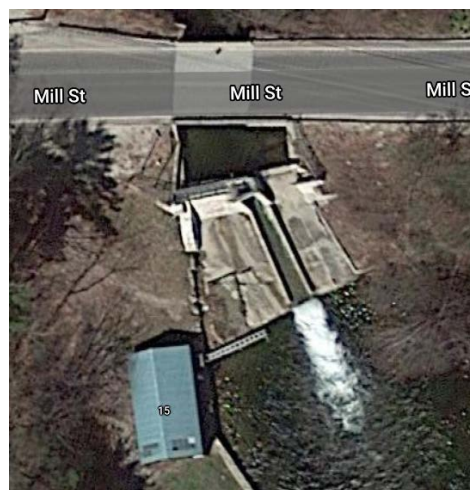
Panther Pond Dam, a significant hazard dam, beside U.S. Route 302, with flooding potential.
