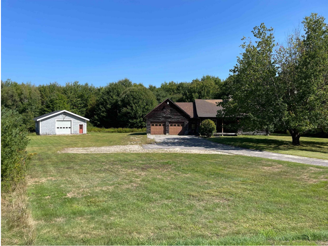
Residential home 173 Cumberland Ave, North Yarmouth. September 8, 2022.
