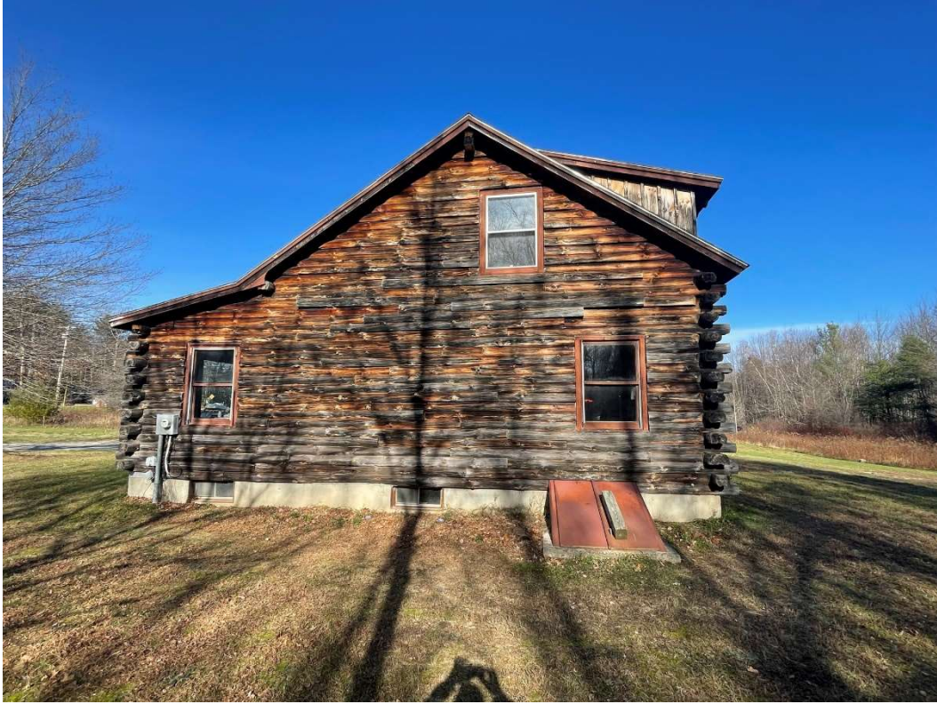
Photo 5 – Building South Elevation
