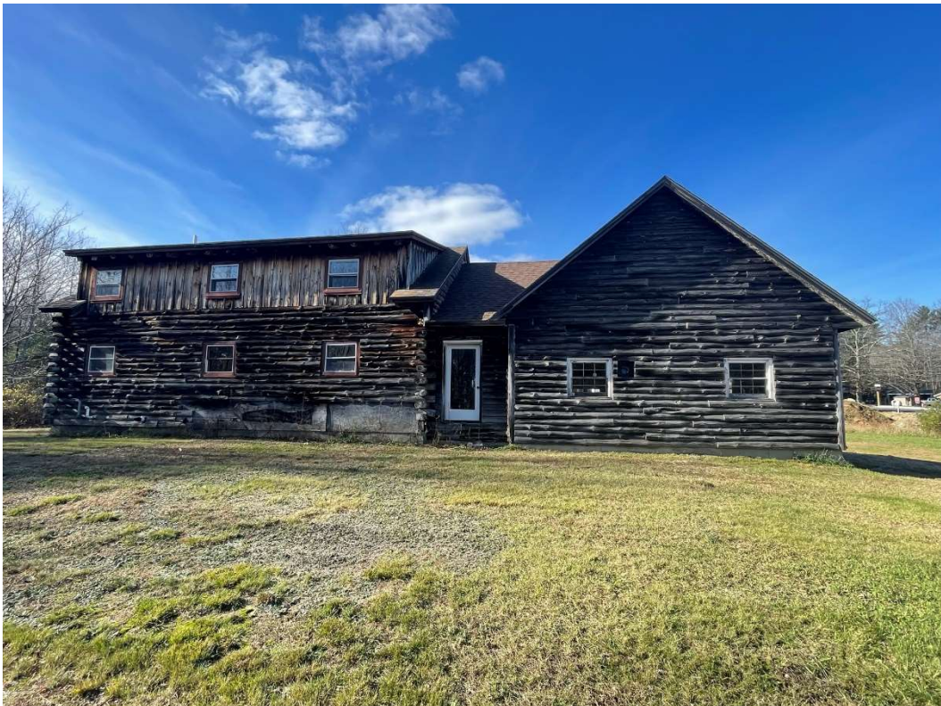
Photo 4 – Building East Elevation
