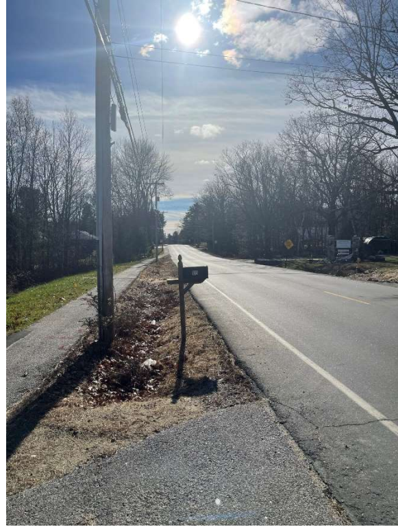
Photo 2 – Looking south along Route 9
