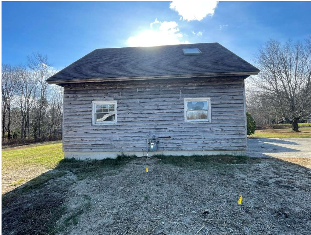
Photo 2 – Building North Elevation
