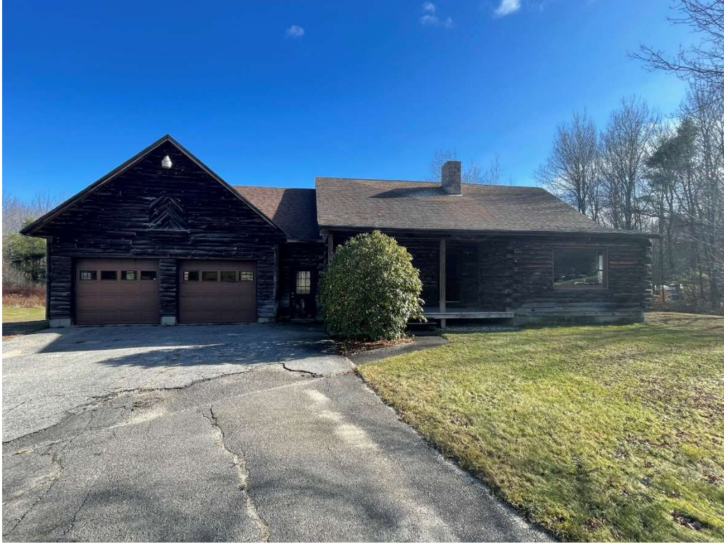
Photo 1 – Building West Elevation
