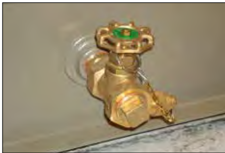
Figure 3. Drain valve with sampler.
