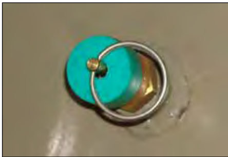
Figure 4. Automatic Pressure relief valve.
