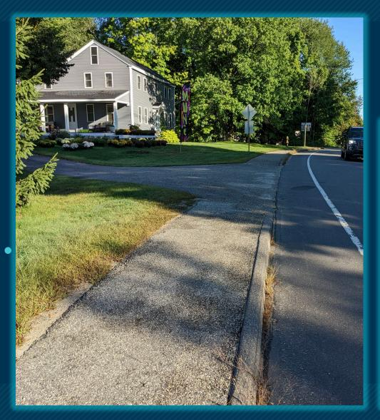
Sidewalk directly adjacent to traveled way-would typically have some closed drainage required.
