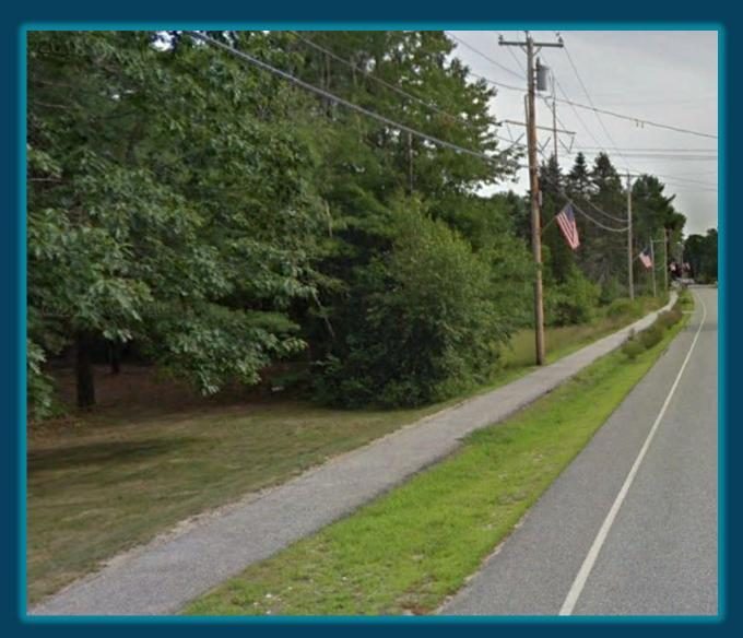
Sidewalk with shallow drainage ditch between walkway and travel surface
