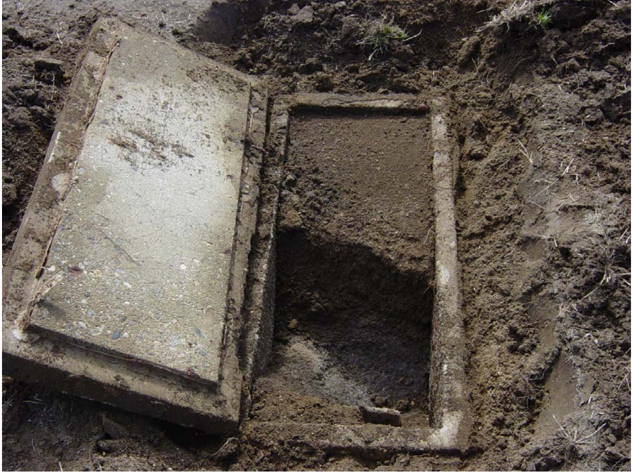
DISTRIBUTION BOX 1 (CLOSEST TO DOSING TANK) NOTE SAND IN BOX
